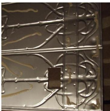
Mark and cut out holes for power outlets, this can be done using the angle grinder.
